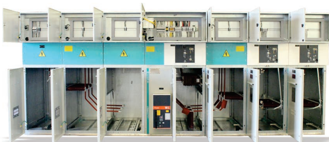
Internal front view
