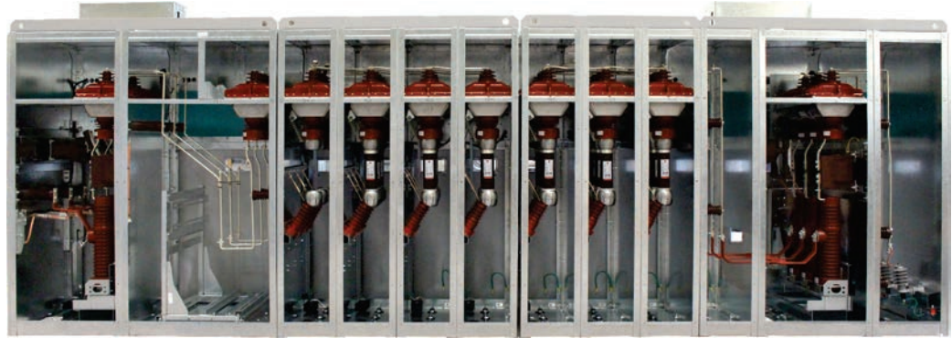
Internal rear view
